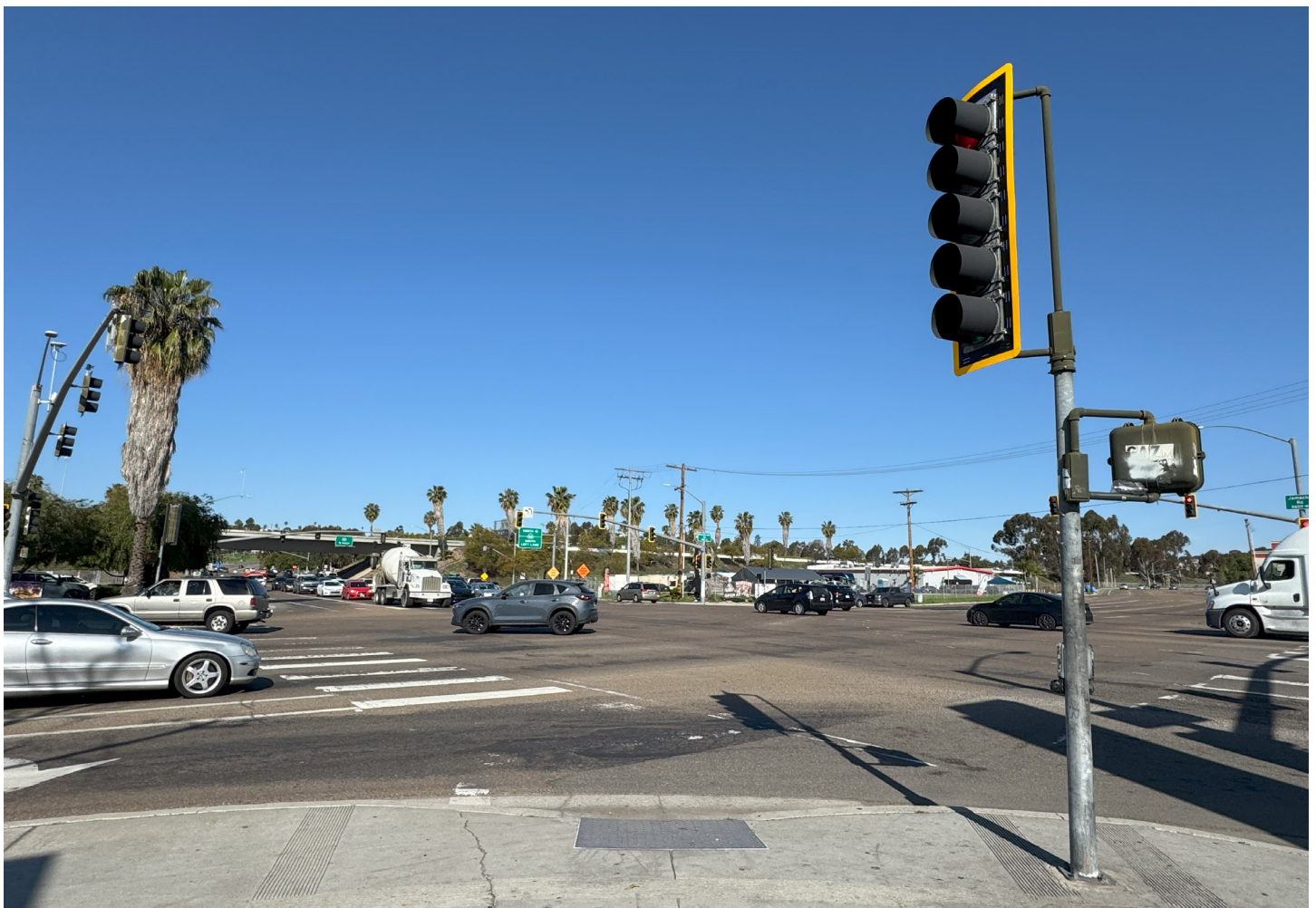
Wide & busy intersection (Jamacha Road and Sweetwater Road) with faded crosswalks
